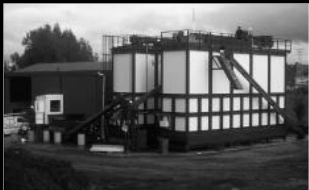
A vertical closed vessel compost unit in Waitakere, New Zealand. Waitakere is a town of 80,000 households within the Auckland region. The unit has a capacity of 14,000 tonnes a year, using ten chambers, which allows different qualities of feedstock to be processed separately.
